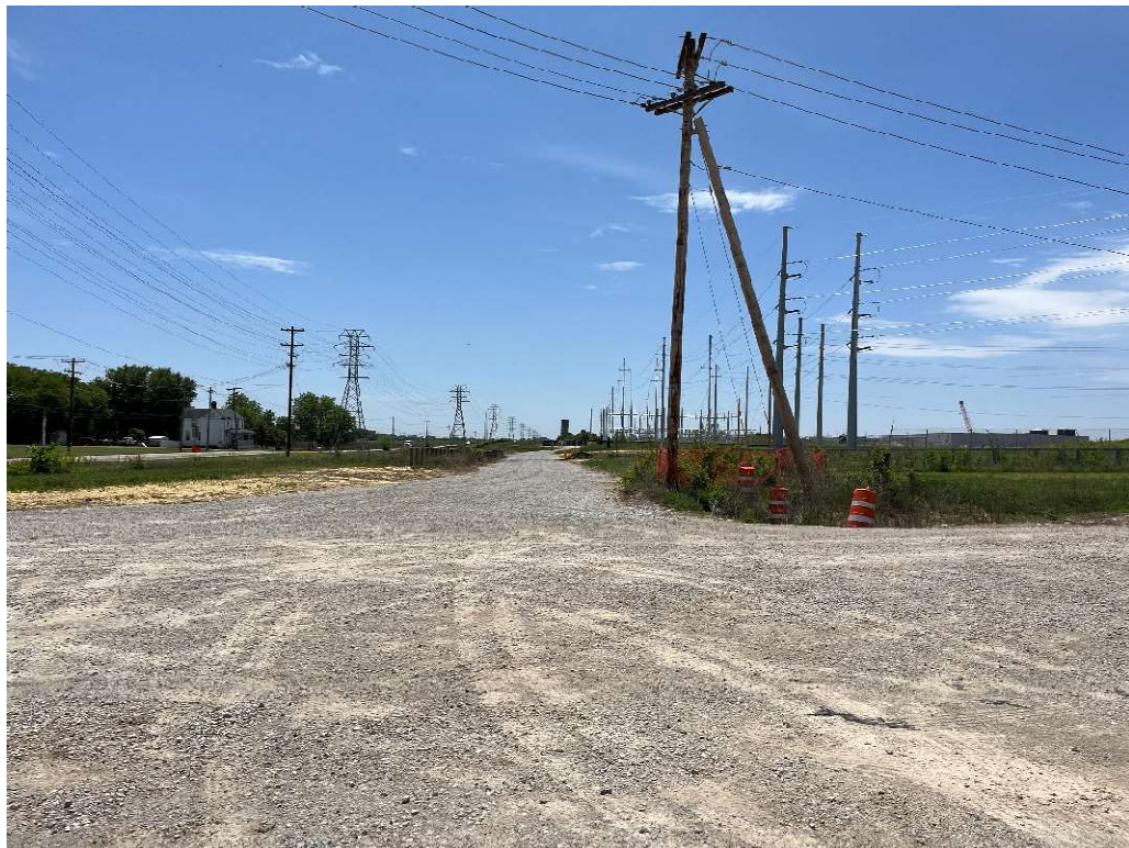
Representative view of the ESC, facing west during the May 25, 2023 environmental survey.
