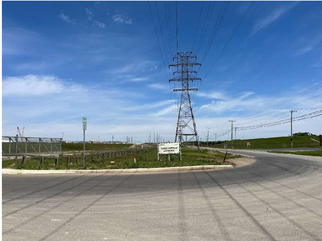
Representative view of the ESC, facing north during the May 25, 2023 environmental survey.
